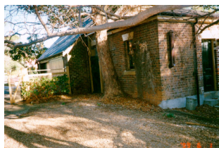
Figures 37 and 38. Whether purpose planted or self-sown, this tree is obviously causing damage to the adjoining building (above and below).
