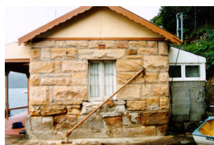
Figures 44 and 45. Inappropriate cement-rich repointing and rendering to this stone building (above and below) has probably been done in response to a breakdown in the original lime based mortar. This is a classic example of what not to do. Cement rendering is not the answer to rising damp as it only pushes the damage higher up the wall.
