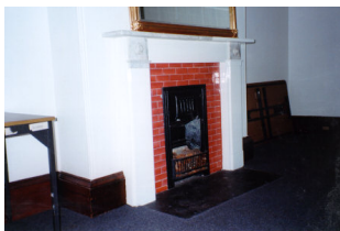
Figure 32. Original elements of this fireplace, in particular the marble pieces incorporated into the reconstructed chimney piece were found behind the covered fireplace opening during conservation of the house.
