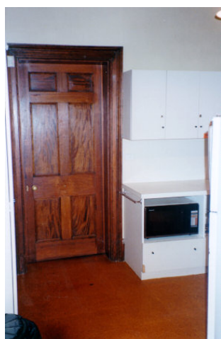
Figure 25. A modern kitchen was installed in this 1830s house. Note that original walls have been carefully covered by laminated sheet which allows for easily cleaned surfaces, but can be reversible such that intervention to original fabric is minimal
