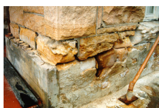
Figures 44 and 45. Inappropriate cement-rich repointing and rendering to this stone building (above and below) has probably been done in response to a breakdown in the original lime based mortar. This is a classic example of what not to do. Cement rendering is not the answer to rising damp as it only pushes the damage higher up the wall.
