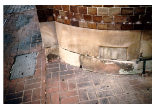
Figure 29. Damp proof course installation should only be considered after exploring all other possible causes of rising damp. This example of a chemically injected dampcourse is used to illustrate the technique rather than the unacceptable manner of patch repair
