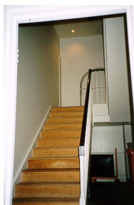
Figure 9. New stair at Hyde Park Barracks
