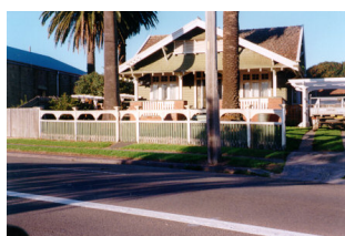
Figure 33. While the base of this significant picket fence needs repair, epoxy patching and painting of existing fabric can be used to preserve most of the significant elements without need for replacement.
