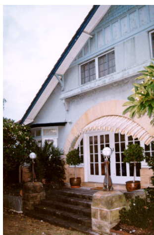
Figure 30. Sensitive design in traditional materials and details allows this porch opening to be enclosed and for more flexible use of the space internally.
