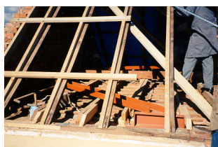
Figure 6. Supplementary roof timbers at Glenmore, Mulgoa
