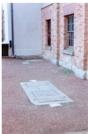
Figure 28. This under-ground grease arrestor was installed next to the Hyde Park Barracks café with minimal intervention to significant interior fabric or archaeological deposits
