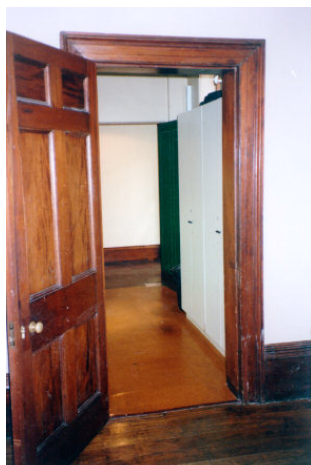
Figure 26. Original joinery, linings, architraves and skirtings have been preserved in adapting this space for a kitchen. New floor covering has been fitted to allow easy cleaning yet original floor boards remain intact
