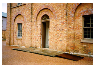
Figure 8. The new entrance ramp at Hyde Park Barracks gives access to the ground floor only
