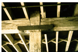
Figure 5. Typical warehouse framing of the 19th century
