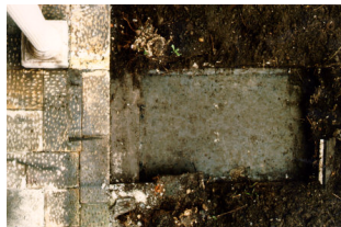
Figures 35 and 36. Historical research and selective excavation uncovered this important remnant of a significant section of paving (above) from which the pathway alignment and design was reconstructed (below)
