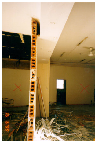
Figure 49. Terracotta lumber used as part of a wall.
