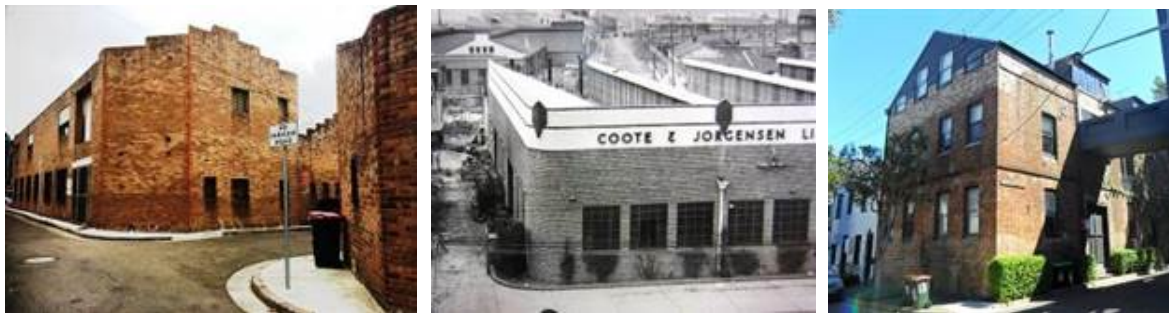
Above: North Alexandria area (left); 602-612 Botany Road, Alexandria (centre); 13-15 Marshall Street, Surry Hills (right)
