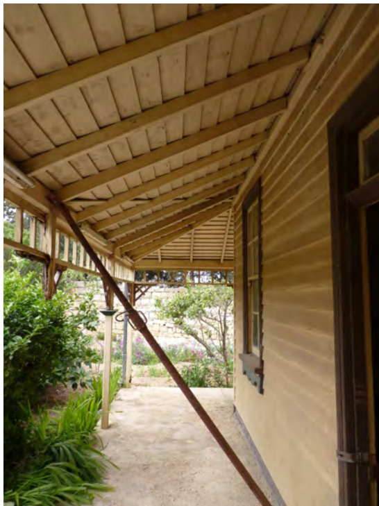
Bungalow verandah, showing props but also timber detailing rare in Malta.
